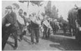
Civilian volunteers going out to dig trenches around Antwerp
